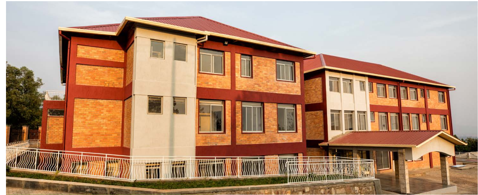
Construction has been completed on the Dream Medical Center with plans for a May 2018 opening.
